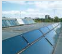
Commercial development Frankfurt, Germany
