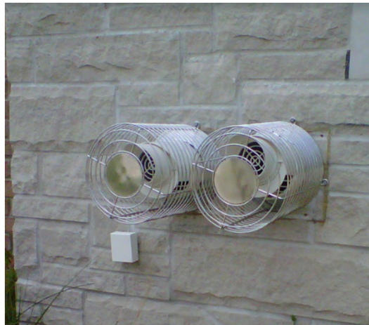
Exhaust and Combustion Air Too Close, even considering prevailing winds
