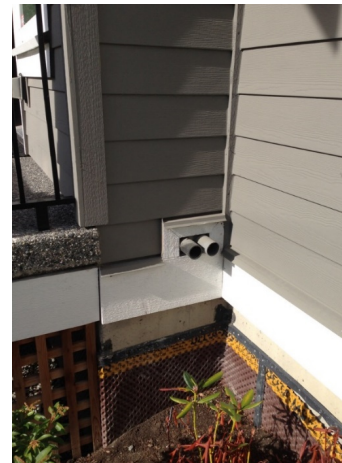
Exhaust and Combustion Air Too Close, even considering prevailing winds
