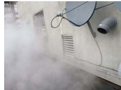
Exhaust and Combustion Air Too Close, even considering prevailing winds
