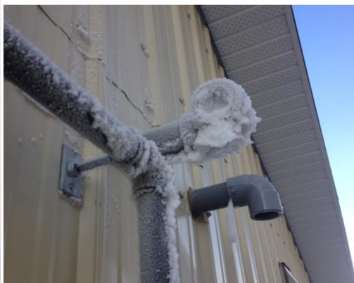
Blockage Due to Ice Buildup/Condensate Restriction
