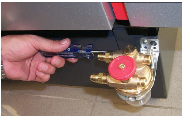
Fig. 9 Mounting filter and check valve assembly
