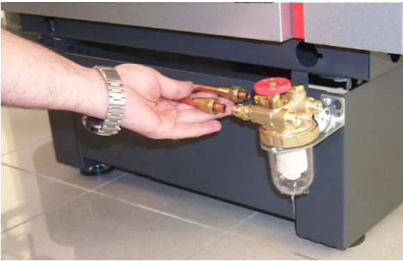
Fig. 10 Connect oil supply and return lines
