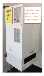
Locate the boiler model on the rating plate.
